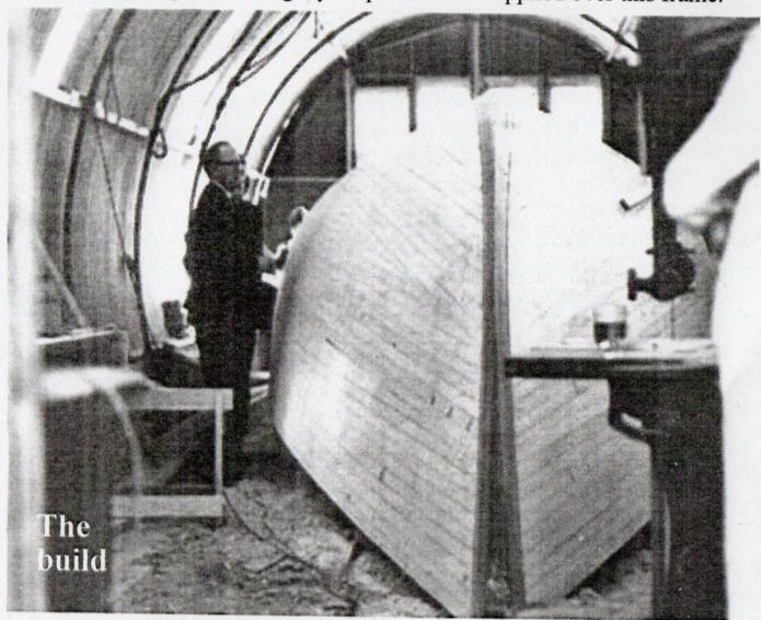
The shell was turned over and the building templates replaced with permanent laminated ribs. A laminated keelson was then laid over them which, with the ribs, added substantially to the strength of the whole structure. Then followed the deck and the engine.
